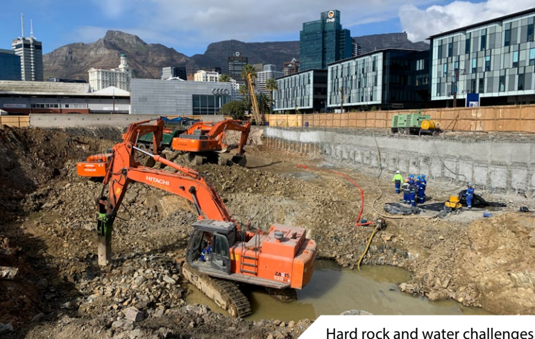
Hard rock and water challenges
