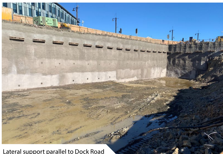
Lateral support parallel to Dock Road
