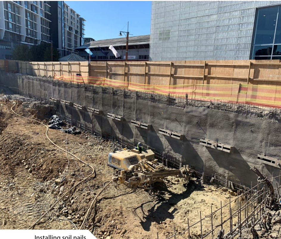
Installing soil nails
