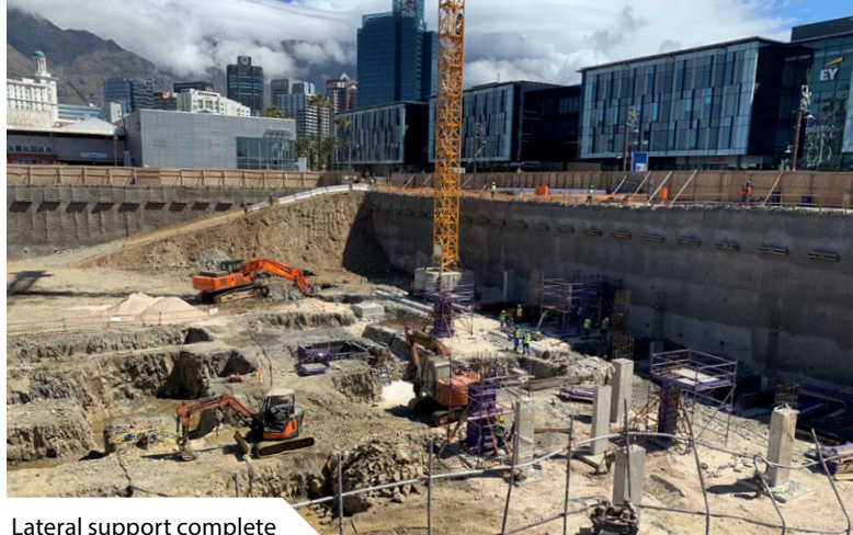
Lateral support complete
