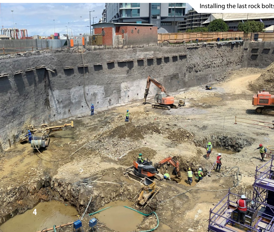
Installing the last rock bolts
