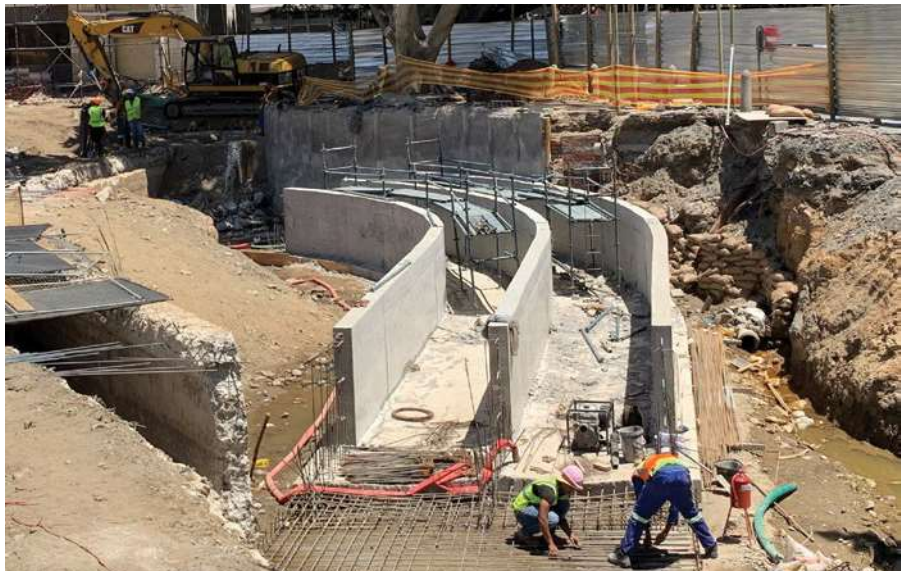
New stormwater culvert with cantilever lateral support in the background supporting the protected tree.
