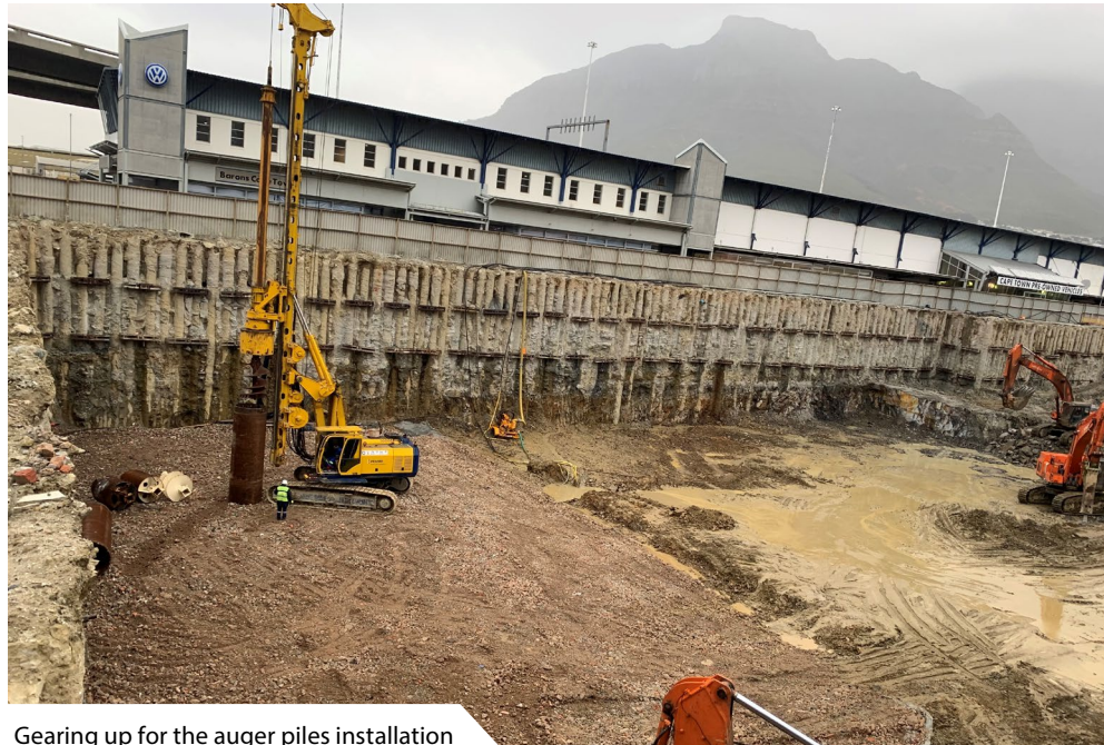
Gearing up for the auger piles installation
