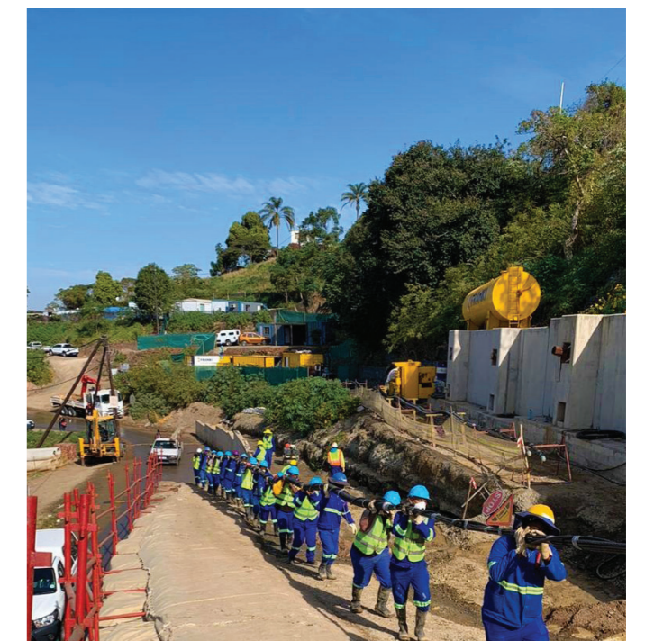
An anchor on its way to be installed.
