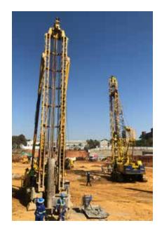
resulting in unstable test pits. The combination of these challenging conditions necessitated the scrutiny of the various piling techniques available and, ultimately, the Franki DCIS pile was determined as the optimum piling solution. This was detailed and discussed at length with the client, DRD D&C JV and the professional team and accepted as the piling alternative to be implemented on the project.
